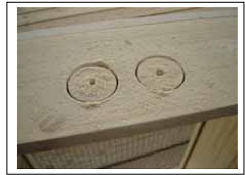
Once both holes are drilled mark a straight line on the outside of the holes to mark what you are going to cut out with the jig saw.
