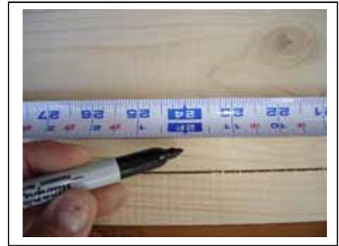
I then took both pieces and measured 24 inches and cut them on a cut-off saw. I again measured 24 inches and cut the boards again so I had 4 pieces of wood 24 inches in length, 2 at 6 inches wide and 2 at 1 inch wide.
