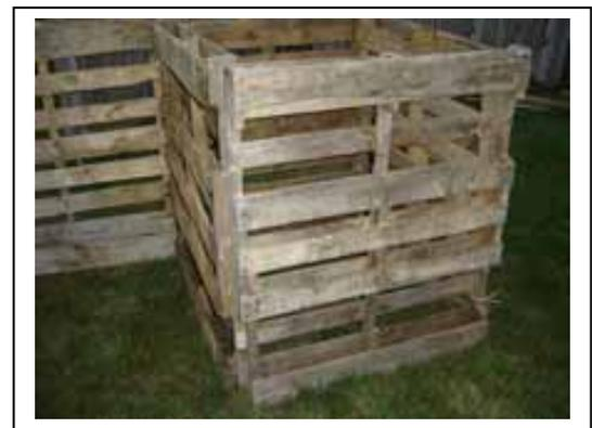
Once you have the first square finished, you can start building your second square. After that, attach the two squares together with either one or two skids to complete the Three Compost Bin System.
