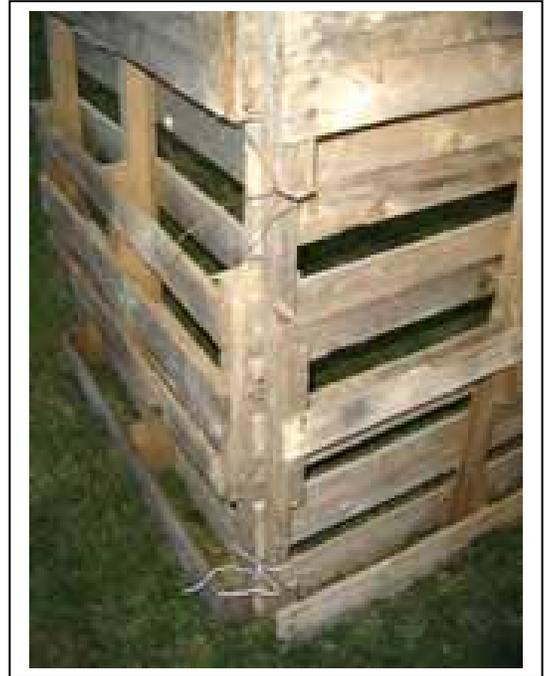
Stand another skid to make a third side and attach it the same way you connected the first two skids using wire at the top and bottom.
