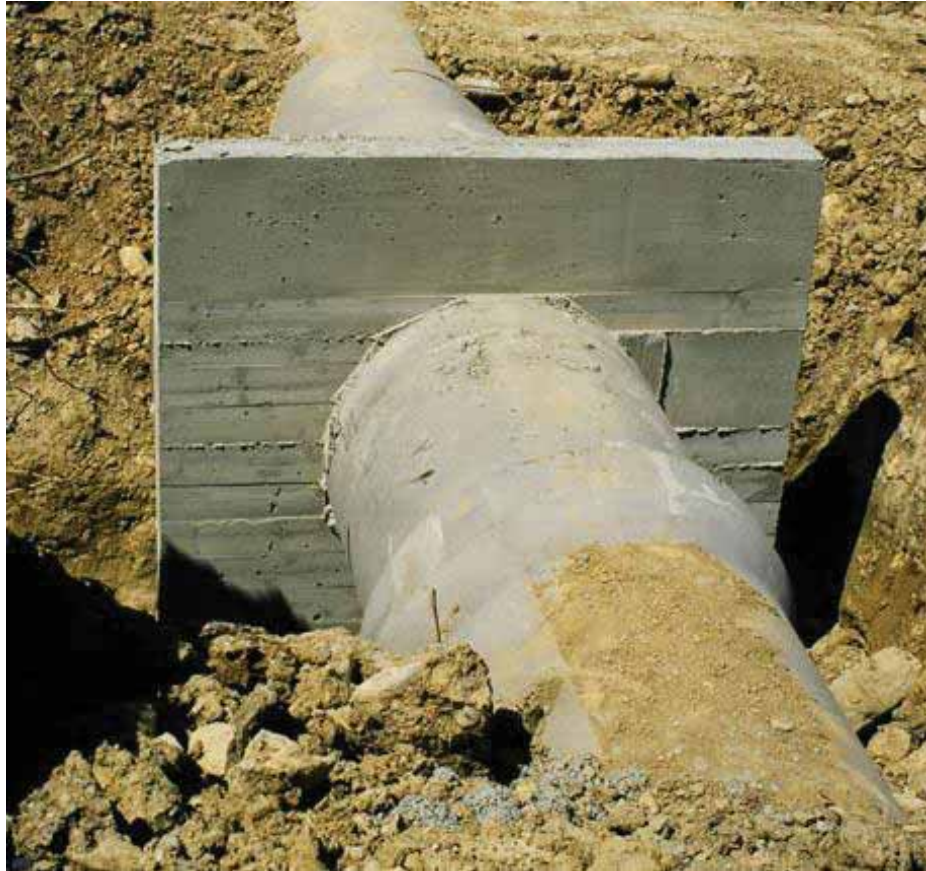
FIGURE 7.6 Anti-seep Collar Design
