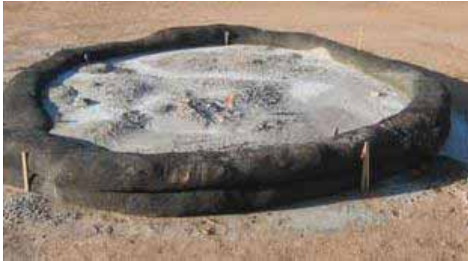
FIGURE 3.18 Typical Compost Sock Washout Installation
